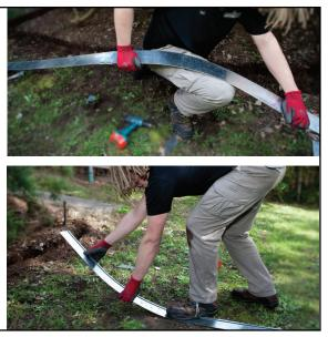
For corners, lay something straight such as a piece of timber, across the edge and lever edging up to create the desired angles. Their are multiple methods of shaping the edging, the best method will depend on the user.
