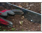
**Tip:** The screw must be under the level of the soil for safety and aesthetic reasons. When using angled stakes, it is necessary to insert two screws at the bottom.
